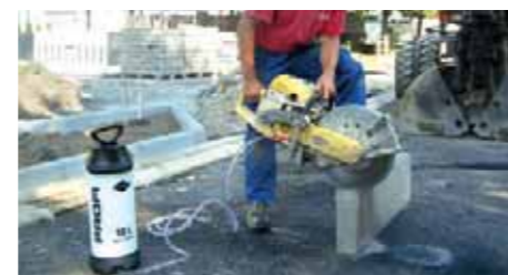
Cut-off grinder in road construction
